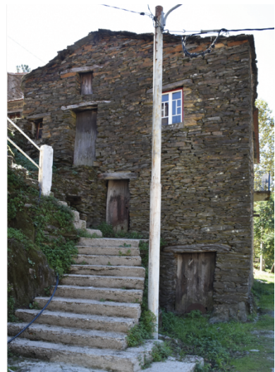
15: Type X house in Fontão, built in schist masonry.
